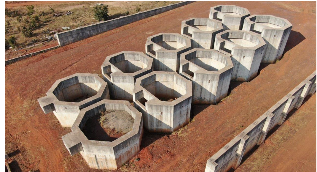
S3 Rougher Flotation Cell Pedestals
