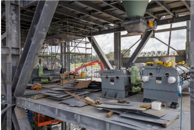
UNIT 1 SILO COAL FEEDERS
