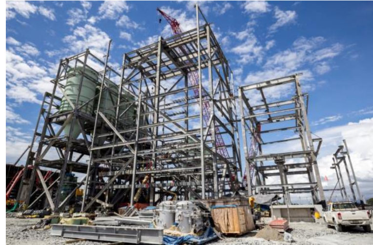
UNIT 1 BOILER & SCR STEEL
