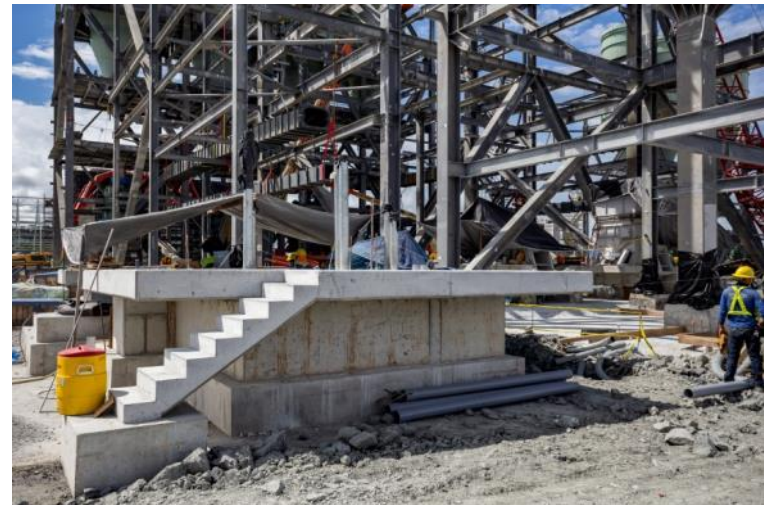
UNIT 1 FD FAN FOUNDATION – EAST SIDE
