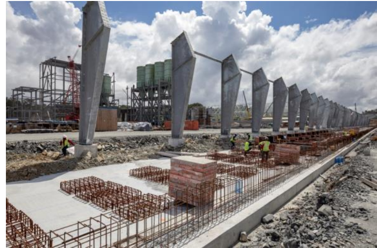
COAL STORAGE – INTERNAL CONVEYOR FOUNDATIONS
