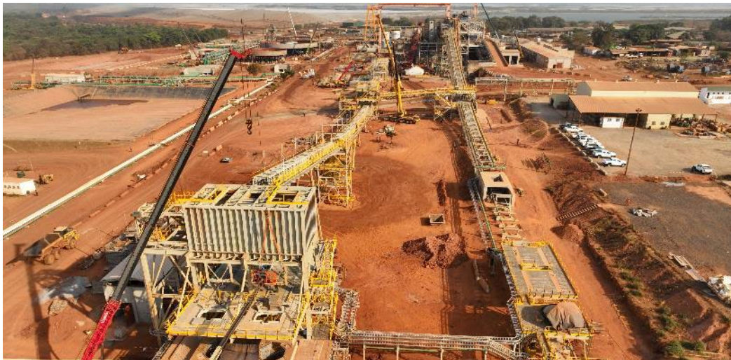
SAG feed and pebble conveyors
