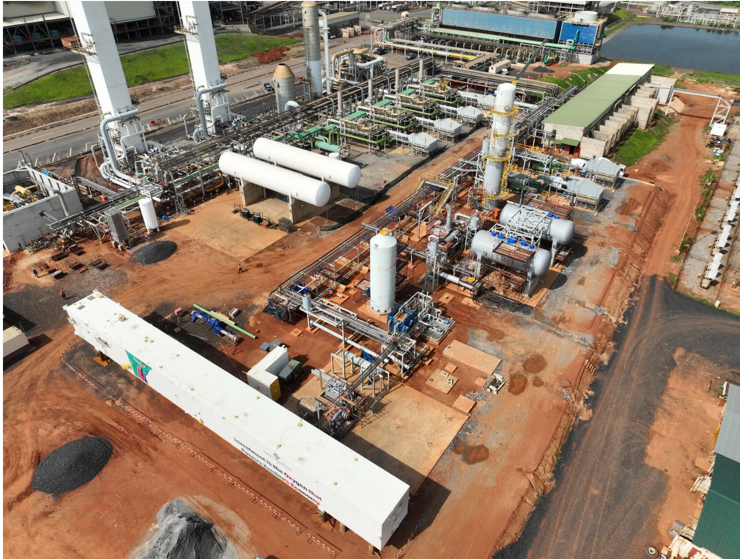
Oxygen Plant Cold Box due to be stood up in Q1 2025
