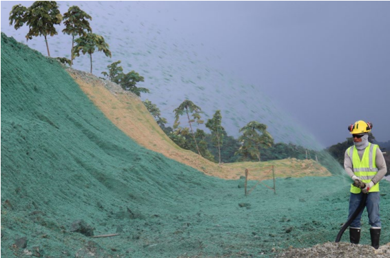
Hydroseeding at Cobre Panamá
