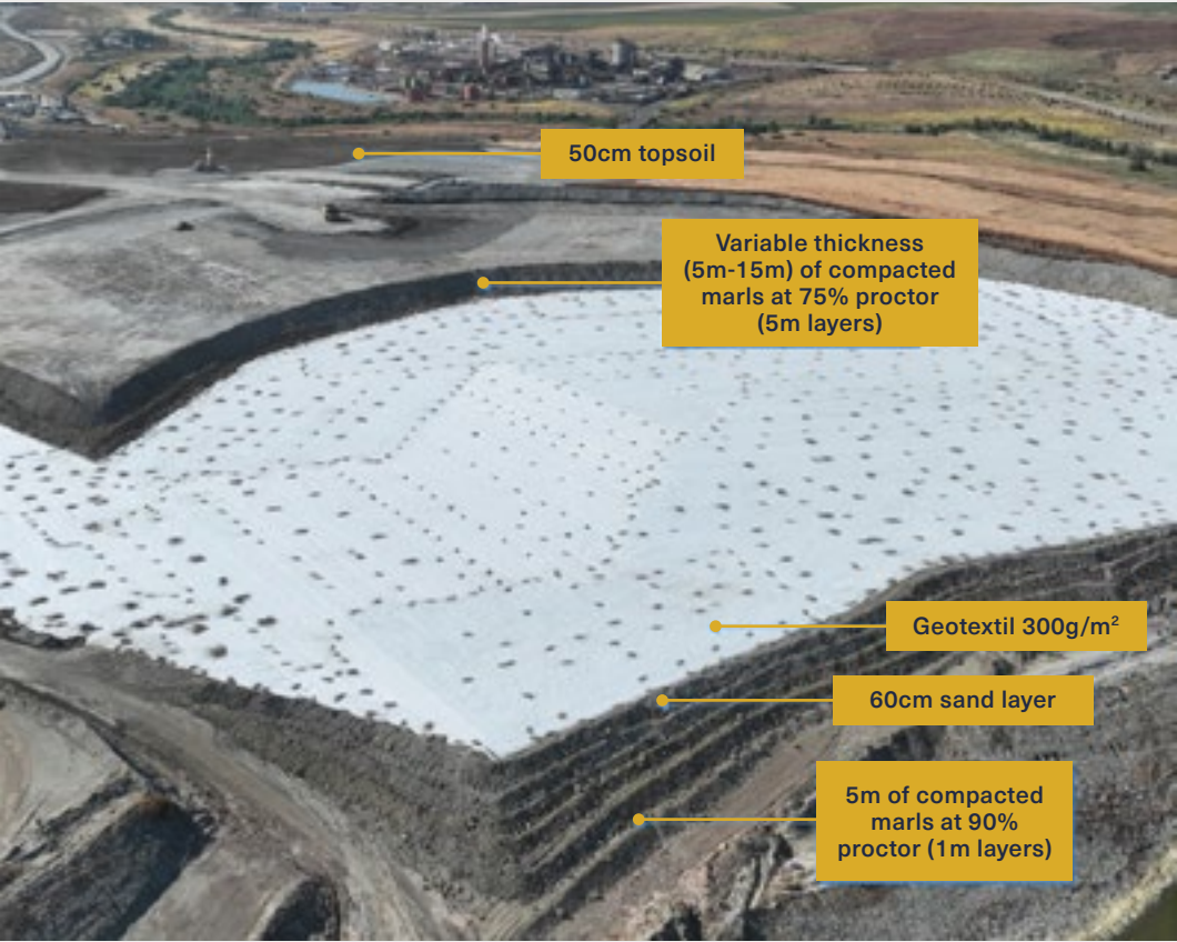
Las Cruces TSF materials profile according to the closure plan.
