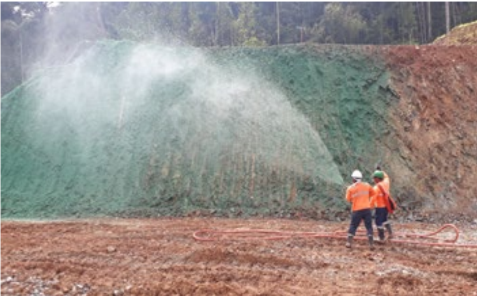
Hydroseeding in Cobre Panamá
