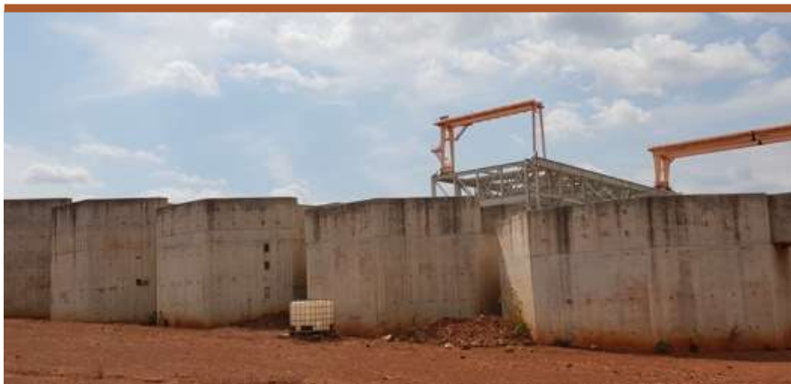
S3 Rougher Flotation Cell Pedestals
