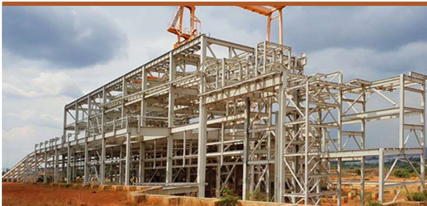
S3 Rougher Flotation Cell Pedestals
