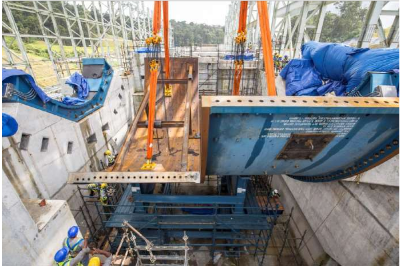
FIRST MILL SHELL INSTALLATION 10-FEB-2016
