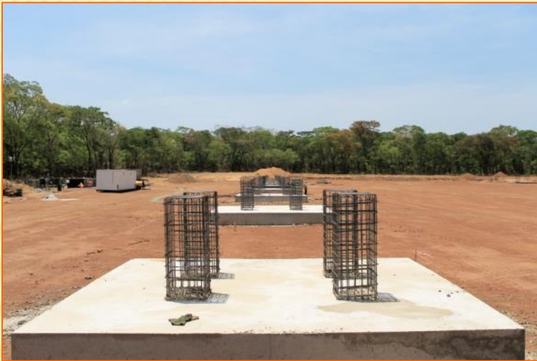
ABB SWITCHYARD, EAST GANTRY FOOTINGS 01-NOV-2013
