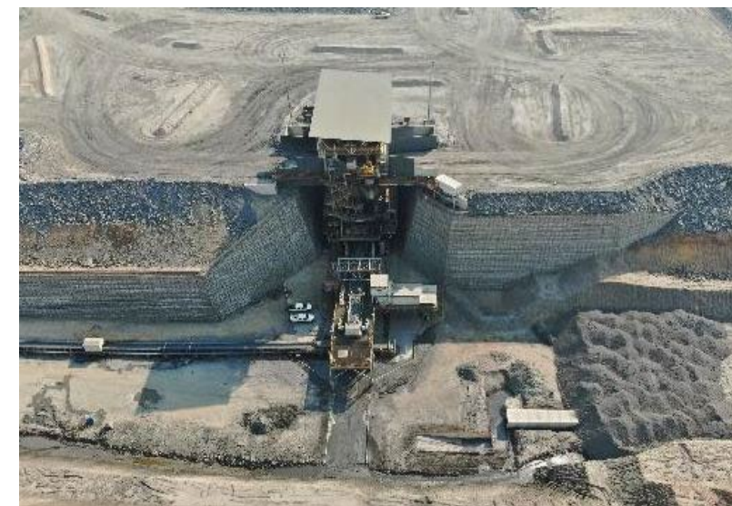
In Pit Crusher in Stage 3
