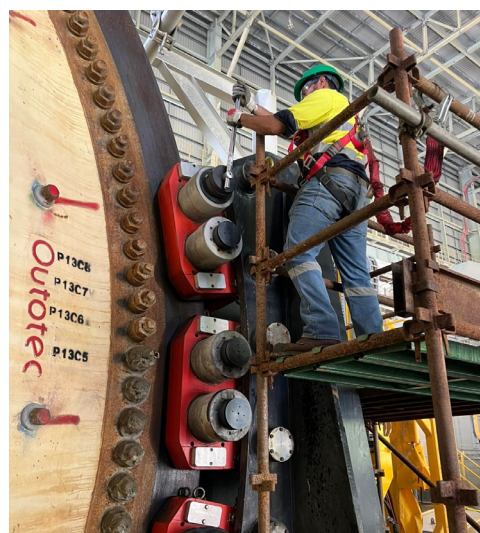
SAG Mill 4 brake maintenance
