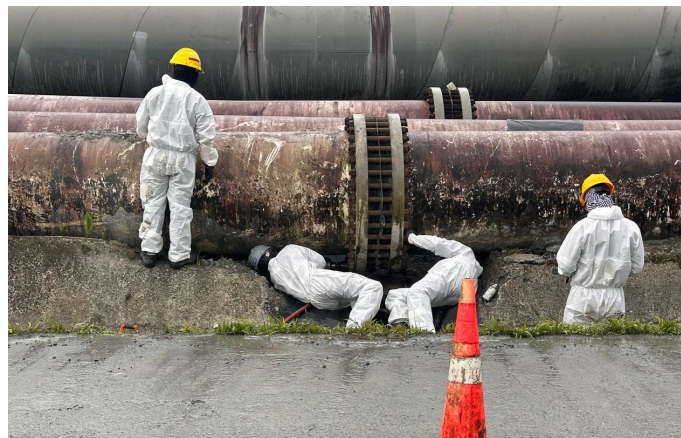
Tailings line – Inspection and bolt replacement
