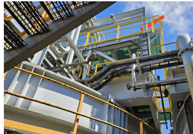
Restored flotation piping supports, process tanks and access platforms
