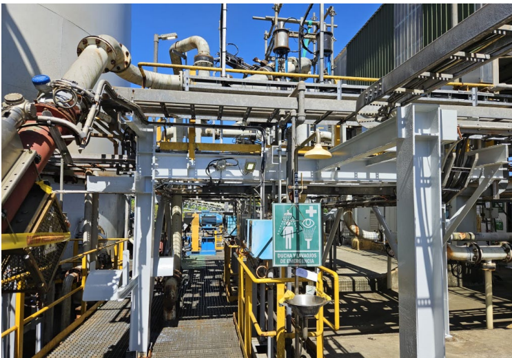
Refurbished concentrate handling area walkways and safety shower stations
